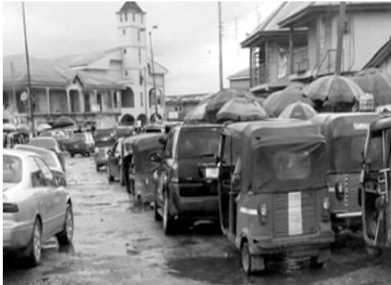
Fig. 3: Asphalt failure, Airport road, Warri
